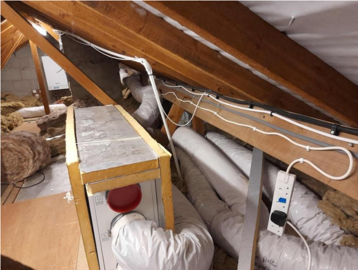
Whole House Ventilation and Heat Recovery Unit + ducting
